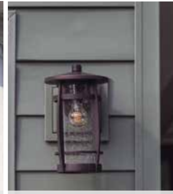
Mounting blocks can be applied in contrasting or matching colors, around outlets and fixtures.
